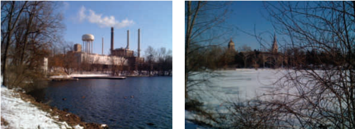
Figure 4.25: St. Joseph's Lake (left) and St. Mary's Lake (right) on the University of Notre Dame campus, 14 February 2010, demonstrating the effect of exchanging heat with the condenser of the Notre Dame power plant near St. Joseph's Lake.
