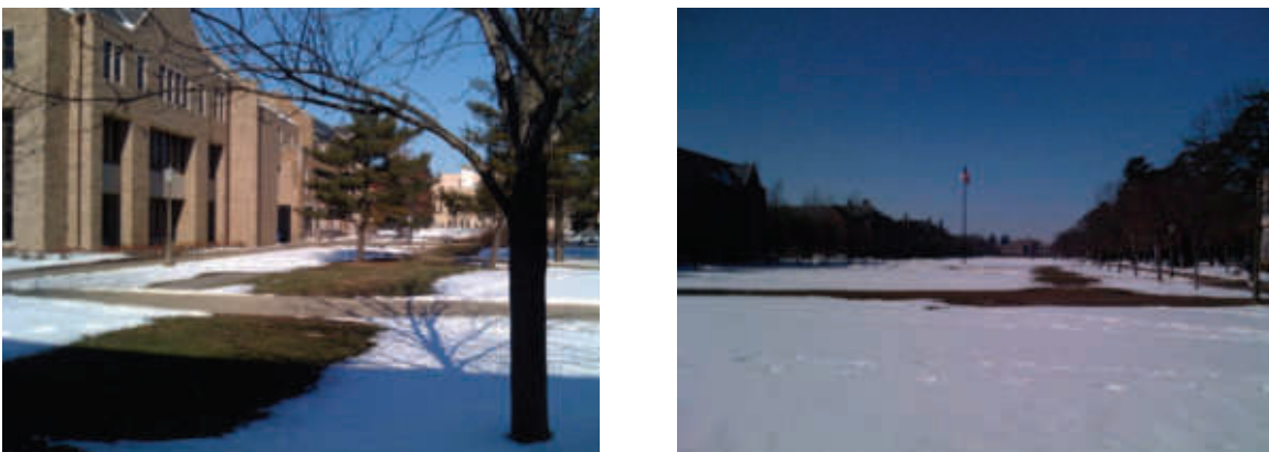
Figure 4.26: Zones of melted snow in regions near underground steam lines on the University of Notre Dame campus, 14 February 2010.
